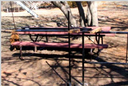
Fence extensions being readied for installation.
