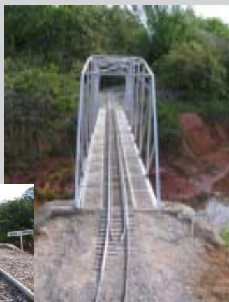
Truman and Harvey worked to install the new track panels on the bridge. Although the old track came off in one section, it could not be put back that way, and each panel had to be put back down one at a time.
